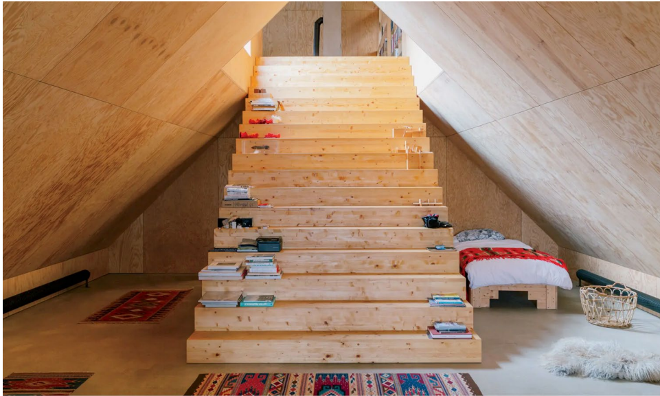
The stairway leading from the second-floor office-lounge to the library and sleeping area on the third floor. Vo decided to use light plywood for the walls and ceiling of this room, as well as for the stairs. Angela Simi
