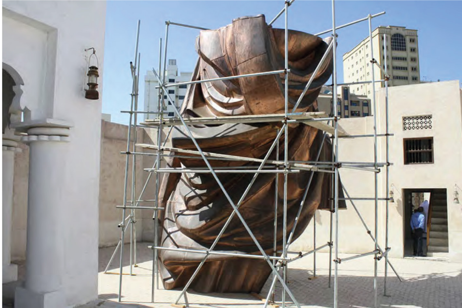
An assembled portion of DANH VO's We the People (2010– ), a 250 piece-by-piece reproduction of the Statue of Liberty in copper repoussé—made in a Chinese factory. Here, 13 pieces form Lady Liberty's left armpit, rising to the level of the structure around it.
